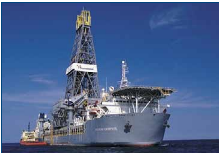
View of the Deepwater Enterprise Drilling rig, equipped with (3) Logan CH clutches in its drawworks, capable of drilling up to 30,000 ft., in 8,500 ft. of water.
