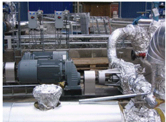
Figure 1: Tuthill Gear Pump Asphalt Installation
