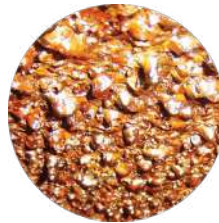
Varnish on reservoir ceiling (Stalactites)
