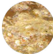
Varnish deposits on reservoir floor (Plated)
